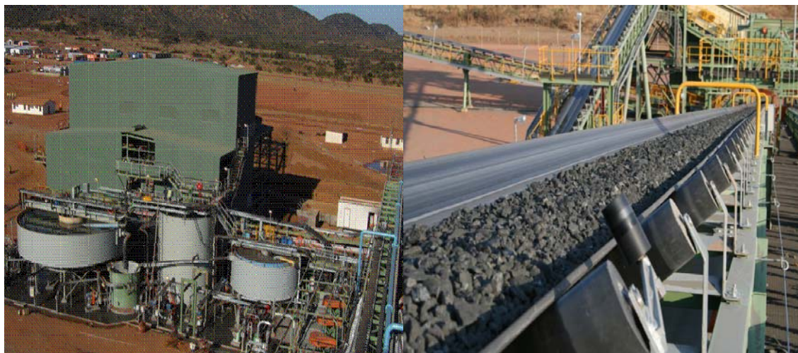
View of float circuit, thickeners and concentrate shed.
